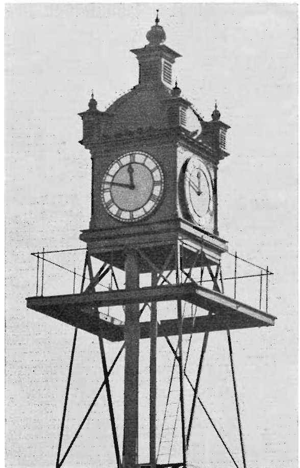
Spencer Street tower clock.
