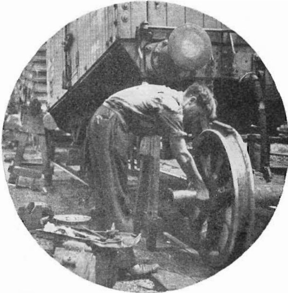
Typical activity in the lifting yard.
