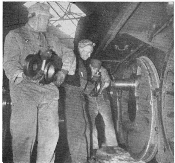
Overhaul of a locomotive in the depot "roundhouse."
