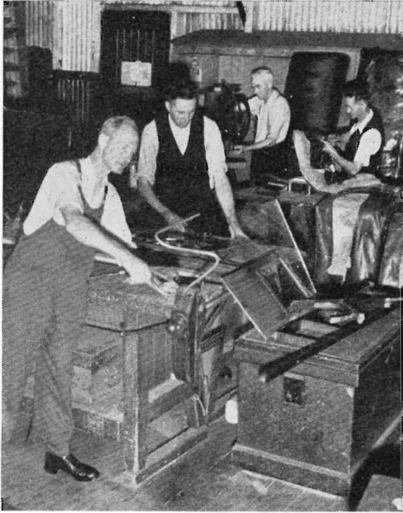
Vandalism, unfortunately all too common, takes up valuable time in repairs.
